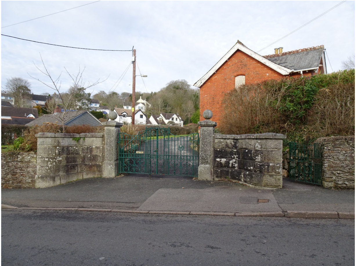
Iron gates with Marshall Trust emblem and granite entrance
