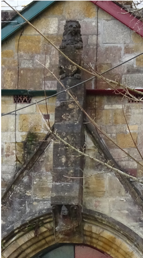
4 of 4 Central porch detail
