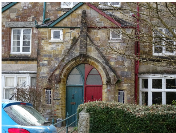
2 of 4 Central porch detail
