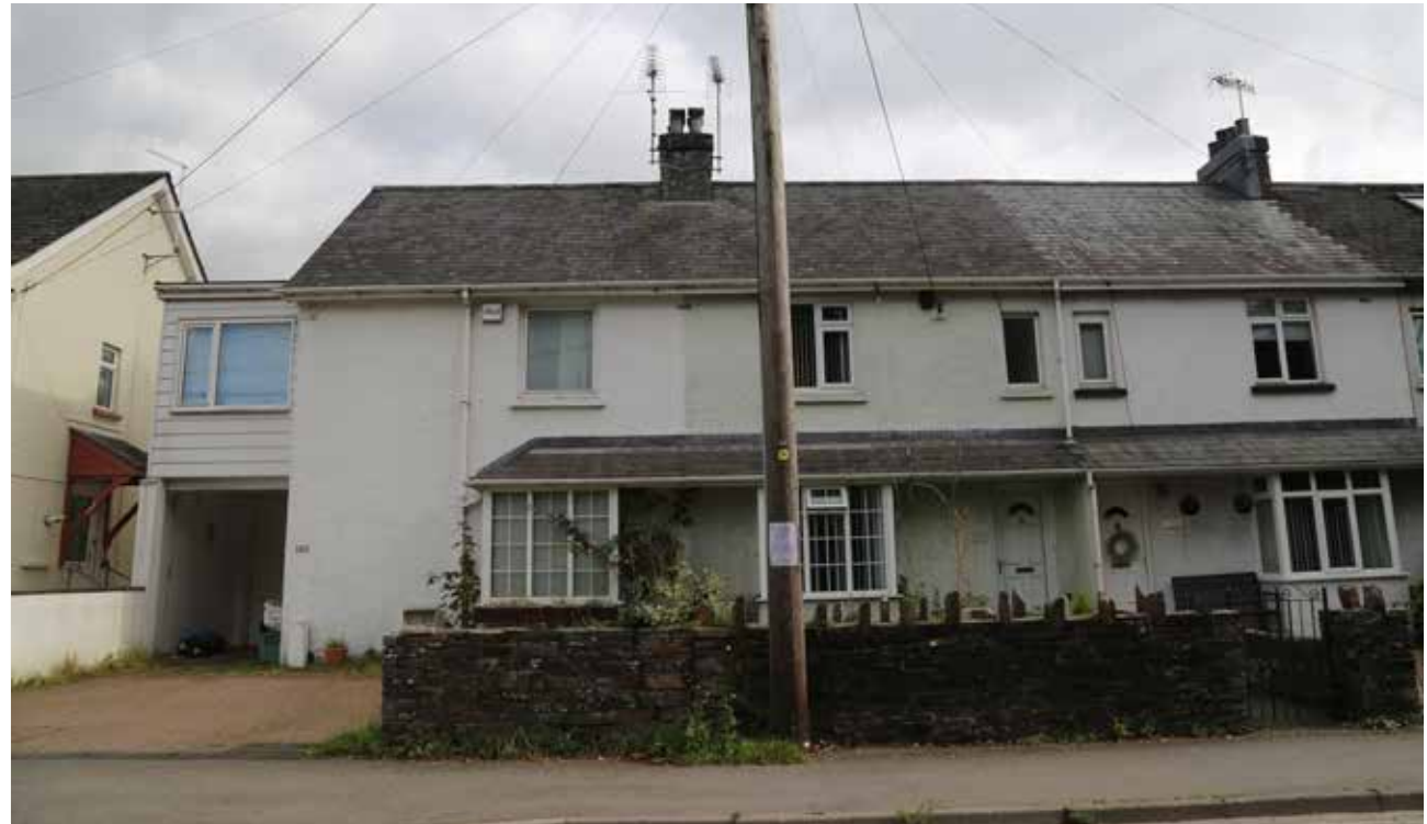
Figure 43: - A386 properties. Low quality flat roofed uPVC clad extension fronting the Conservation Area.
