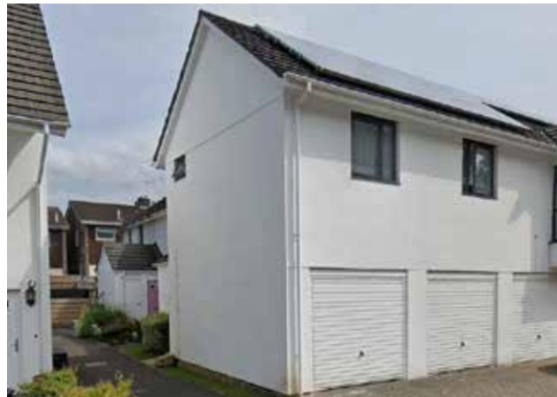
Figure 47: - Flats over garages. PV array on roof.
