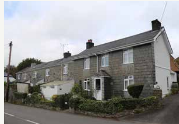
Figure 64: - Example short row terrace, which demonstrates the maximum single development size. Also a good example of slate hanging on the primary elevation.
