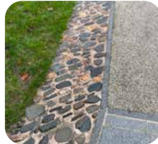
Pebble detail, sympathetic to granite paving and bound gravel
