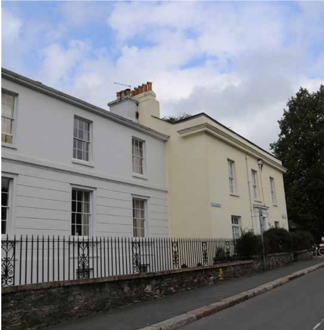
Figure 82: - Granite kerbs, stone wall with capping and railings. Building facades with generous windows and positive fenestration rhythm. Texture and subtlety with string course, plaster work and render detail all in white.
