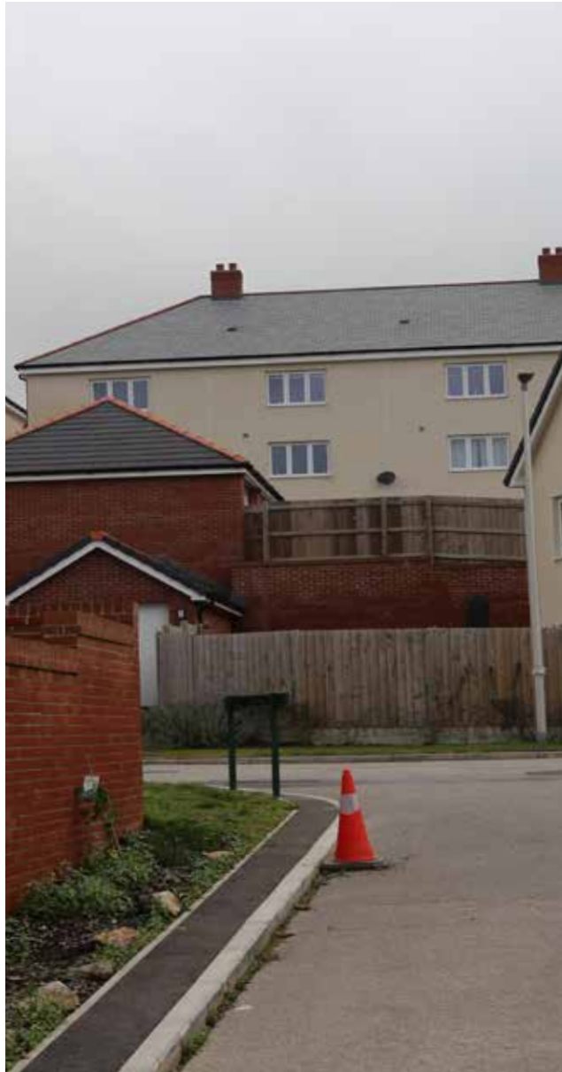
Figure 35: - 3.5m + retaining walls at the rear of recent properties are undesirable.
