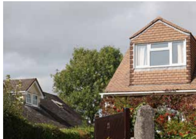
Figure 57: - Two styles of gable dormer, a pitched dormer roof is a more robust detail.
