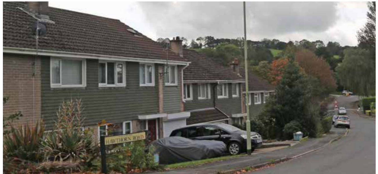
Figure 22: - Tiled panels are likely not cavity constructed and have minimal insulation and therefore more susceptible to elevated heat loss.
