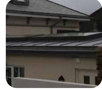
Standing seam with roof light extension roof
