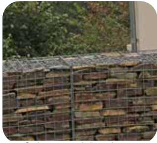
Gabions with local stone
