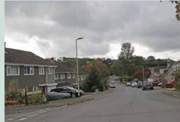
Figure 77: - Plot left susceptible to street water run-off.
