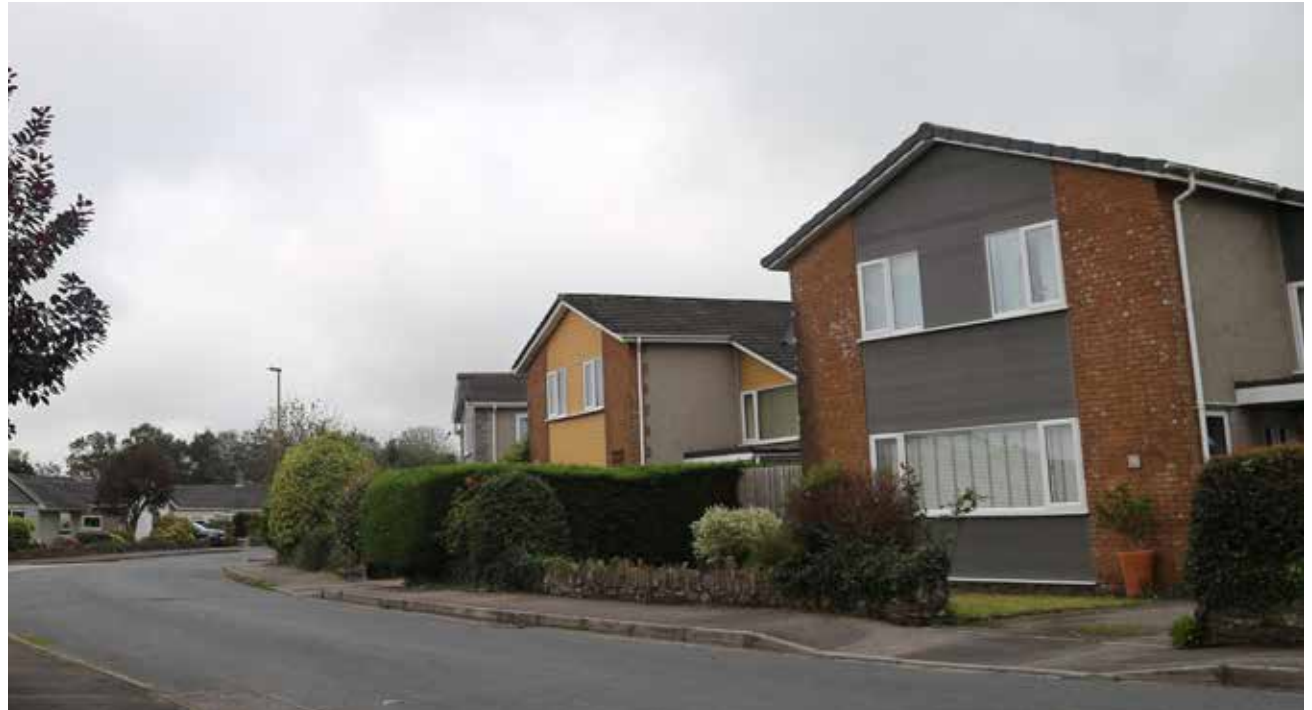
Figure 36: - Examples of material palette. Brown brick, concrete roof, roughcast render and recent composite cladding.
