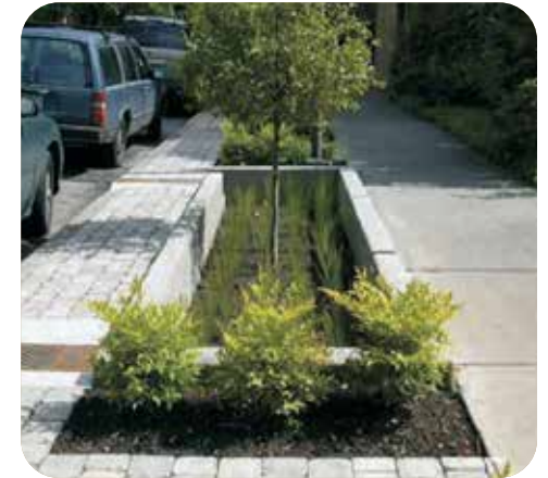
Figure 91: - Rain gardens integrated into pavements provide cross-cutting solutions. (Source:CIRIA).
