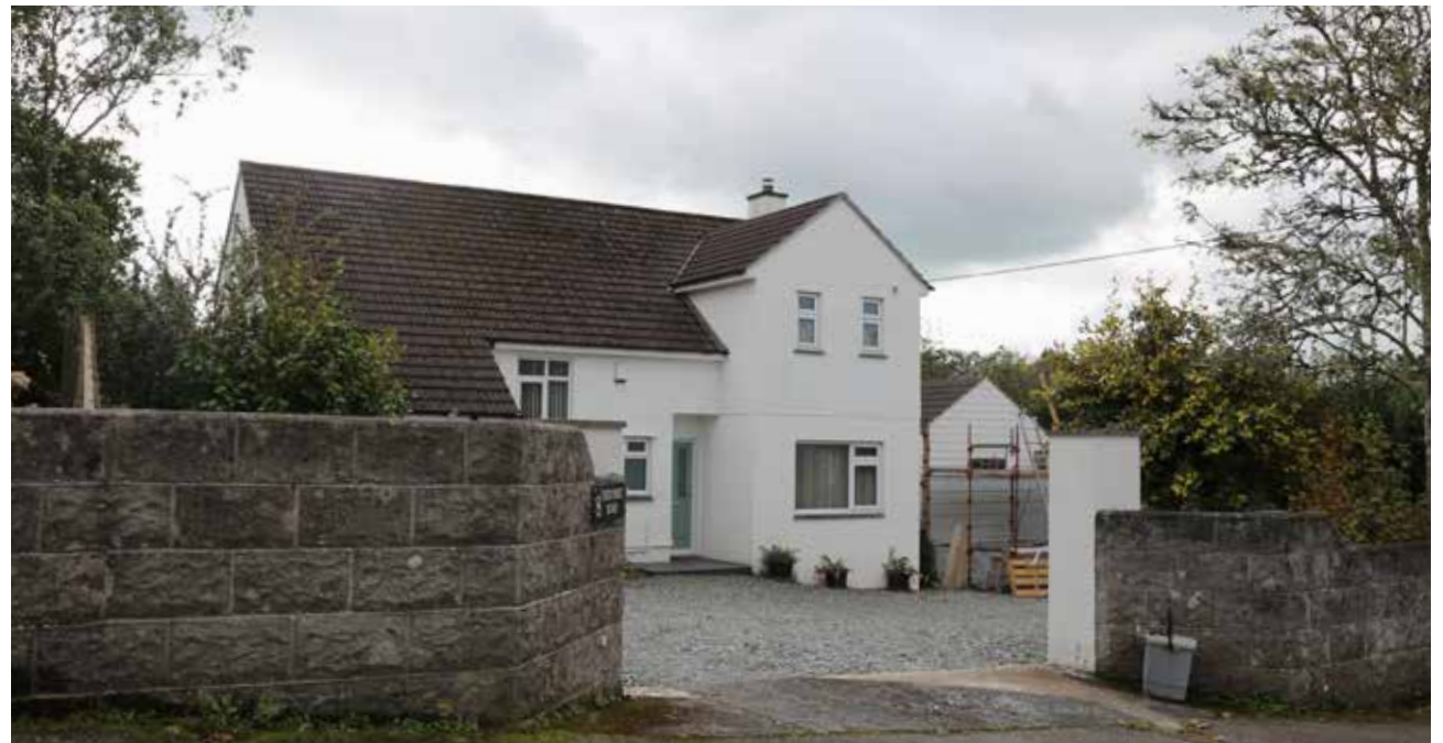
Figure 60: - The storey arrangement can be seen on several dwellings in the Character Area.
