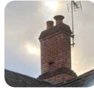
Tall decorative chimneys
