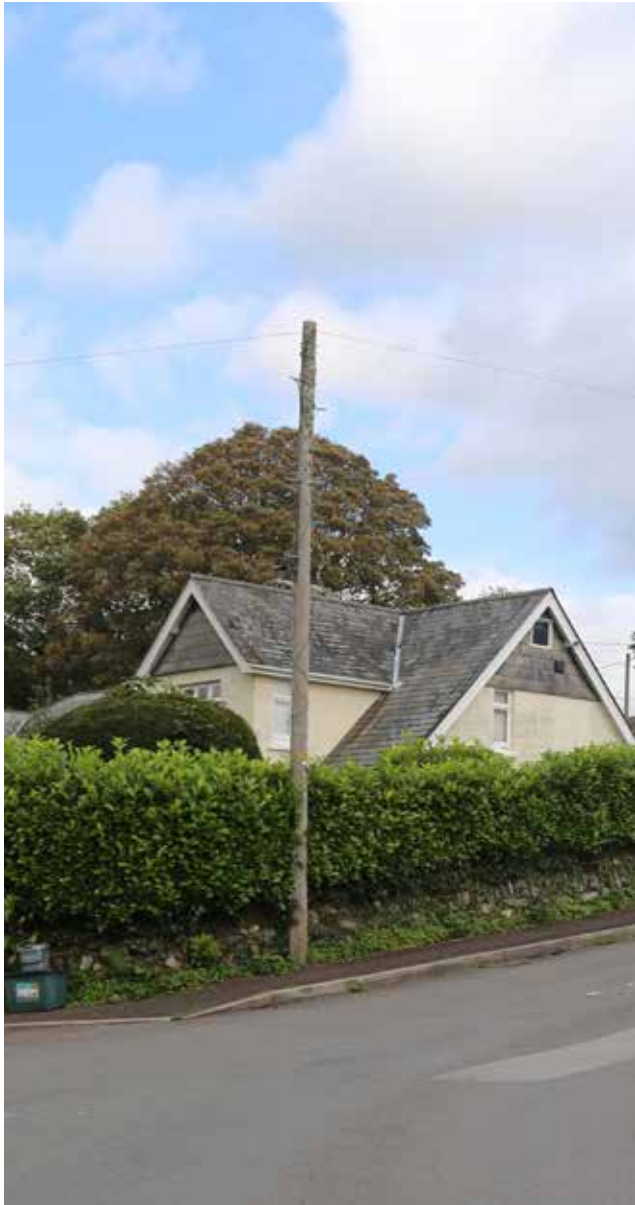
Figure 52: - Slate roof and partial covering a gable. Devon hedge.
