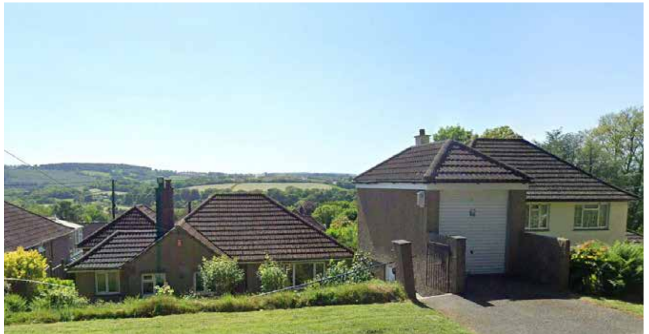
Figure 50: - Response to levels, Whitchurch Road.
