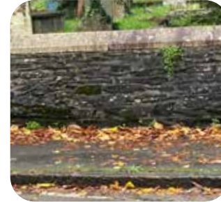
Stone wall granite coping
