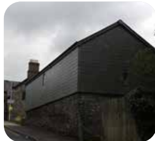
Slate hung upper storey
