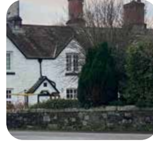
Stone wall, granite coping
