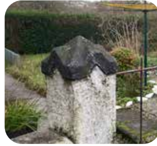
Decorative pier cap
