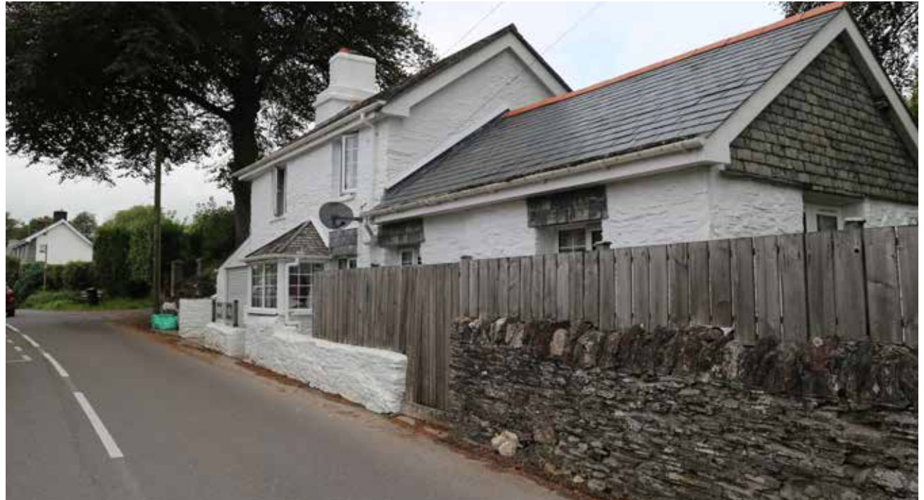
Figure 26: - Stone built house with a textural facade of thinly applied render or whitewash. Quality slate at window heads, gable and porch.
