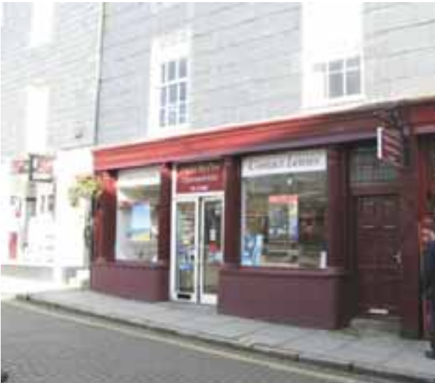
An historic shopfront in Market Street
