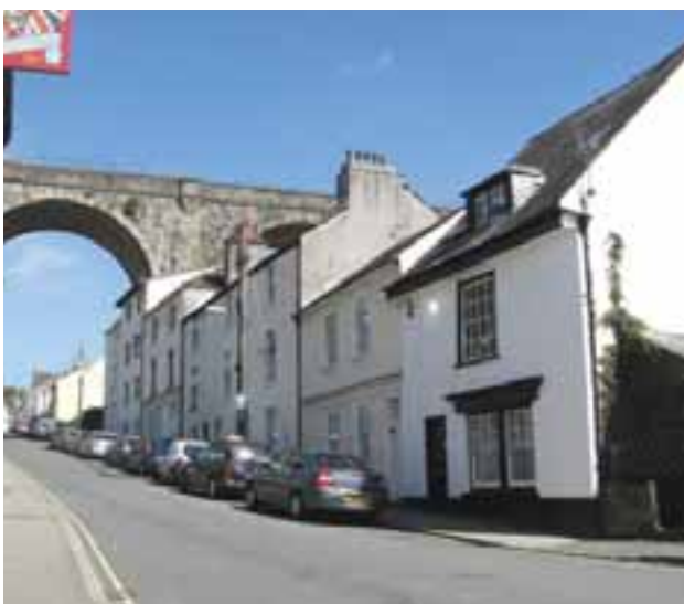
The railway viaduct looking north from King Street
