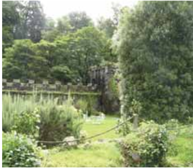
South Precinct wall
