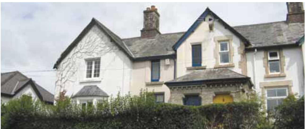
Bedford Cottages in Trelawny Road
