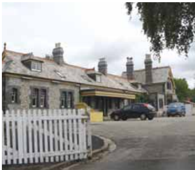
Former Tavistock North Railway Station
