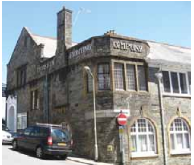
Former Tavistock Printing Company building, Pym Street
