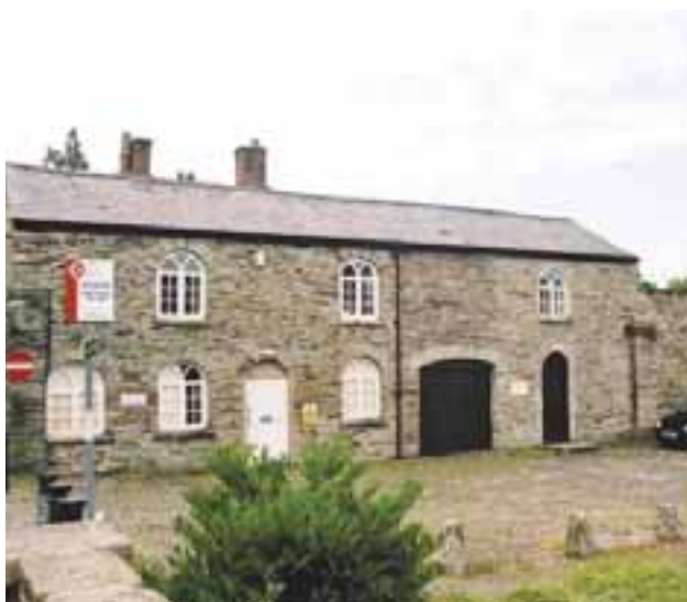
Former canal buildings face the wharf in Canal Road and are used as offices
