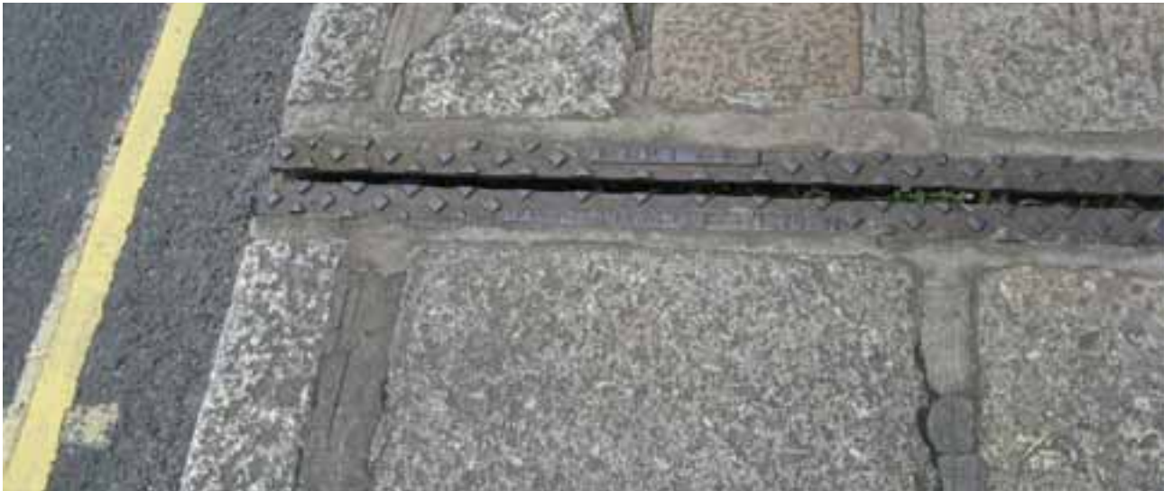
Pavement drain detail in West Street, marked 'Tavy ironworks'
