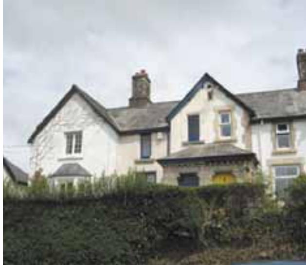
Trelawny Road Cottages
