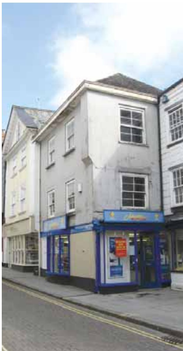
Timber framed building in Market Street
