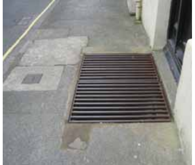
Cast iron pavement grille and granite paving in West Street
