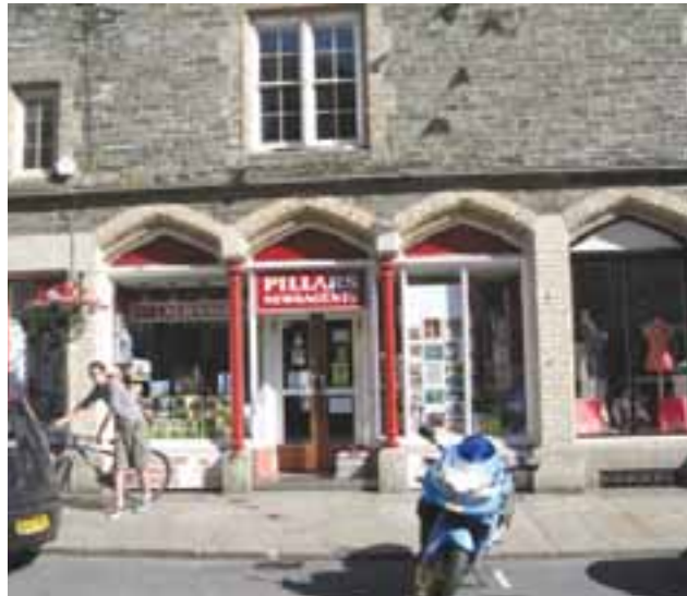
Simple original shopfront facing Duke Street
