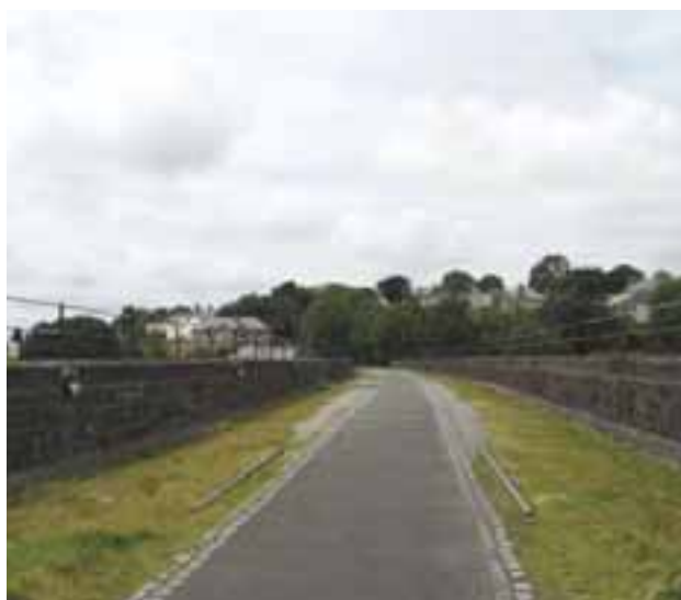
The former railway track over the viaduct is now a public footpath
