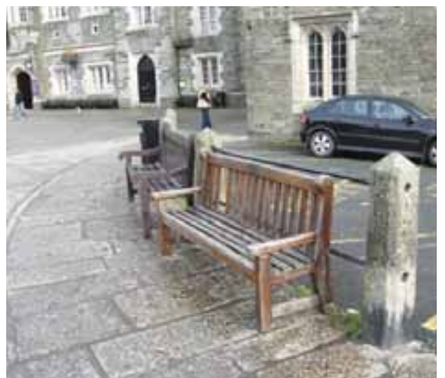
Poor quality public seating in Guildhall Square
