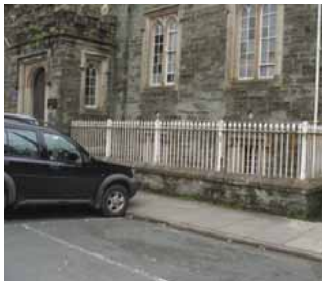
Cast iron railings outside the Guildhall
